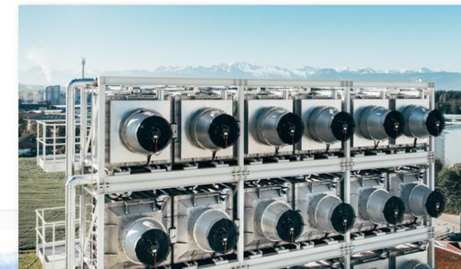
Climeworks' plant for direct air capture in Iceland removes carbon dioxide permanently from the atmosphere. Credit: Julia Dunlop/Climeworks
